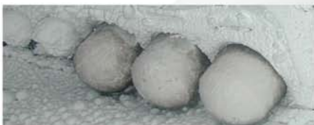
The difference between a wet coated system and a bolt cap system after a fire.
